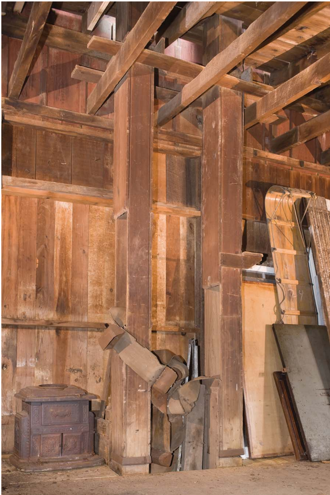
Photograph 19. Detail of grain elevators. View to the northwest.
