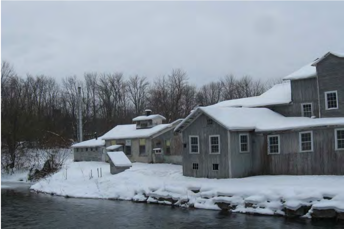
Photograph 7. View of the east face of the mill building/former electroplating facility, with the structural extension that housed the mill waterwheel featured in the center of the photograph. This extension corresponds to section “K” in Figure 4.
