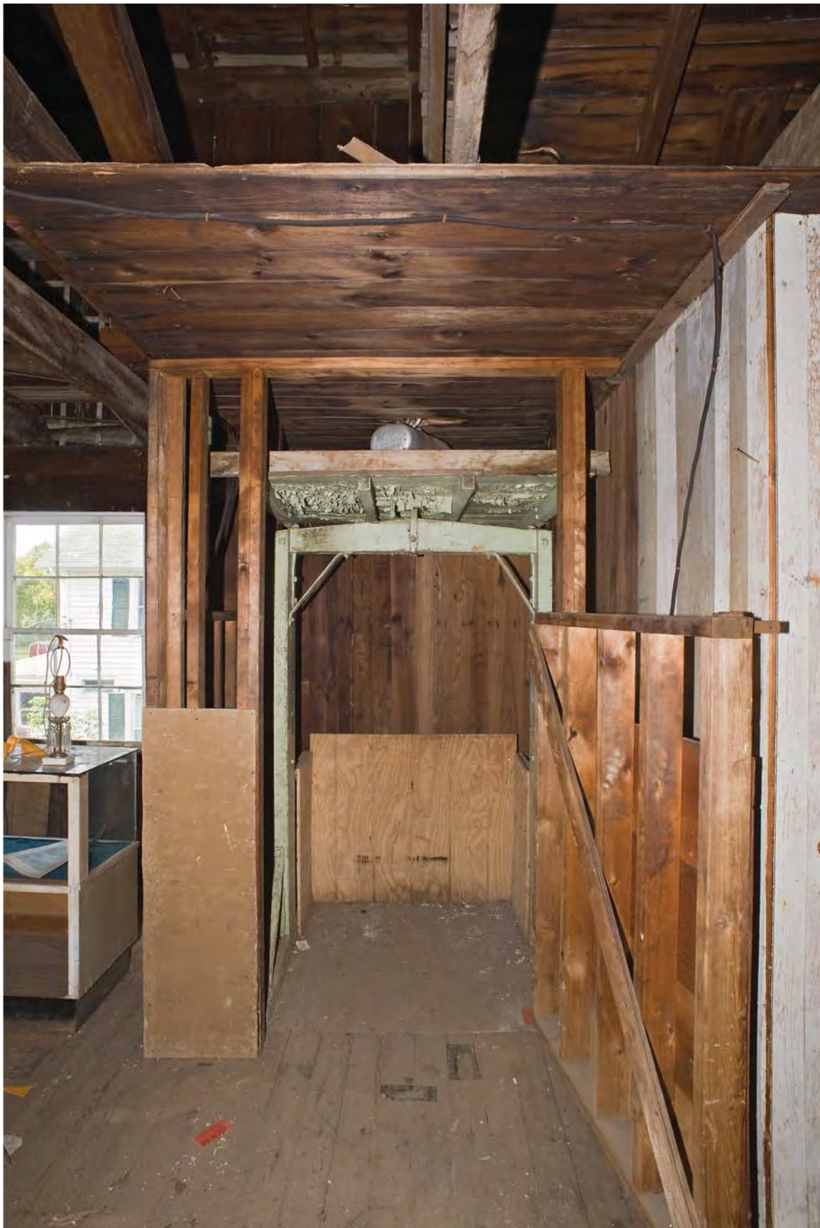
Photograph 23. Elevator, second floor, west side. View to the west.
