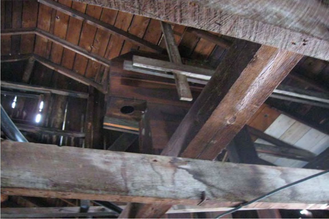
Photograph 11. Another detail of an intact box conveyor used for transporting grain through the mill (located in section "I" in Figure 4).
