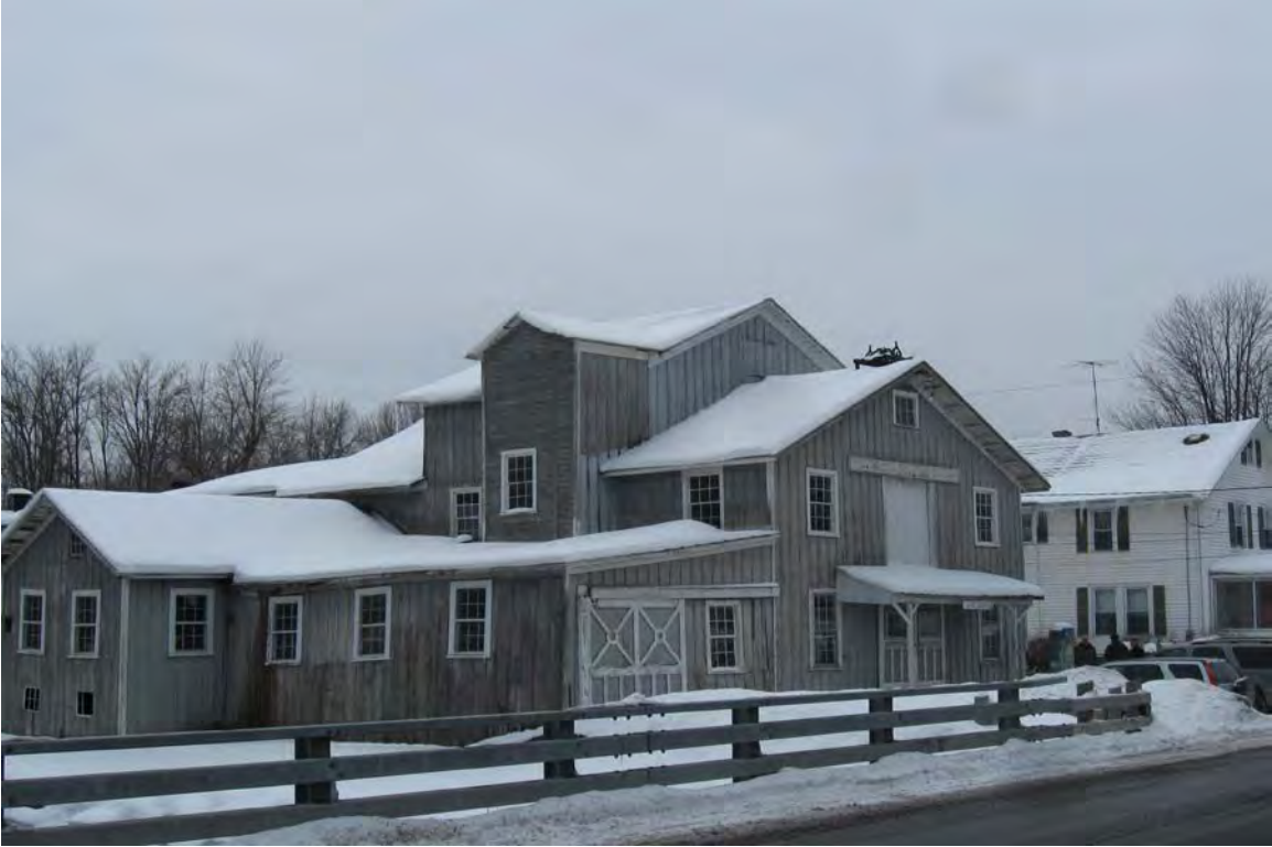
Photograph 1. View of the front and east face of the mill building/former electroplating facility along Green Street. View to the southwest.
