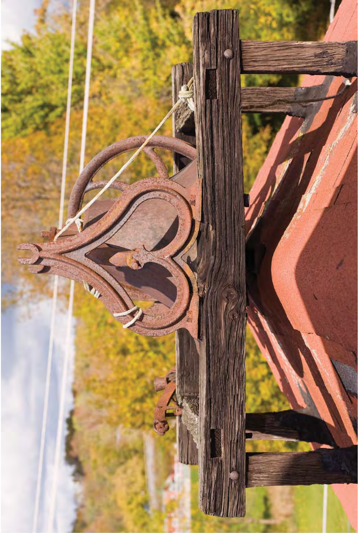
Photograph 14. Bell on front of mill, roof of attic. View to the north.
