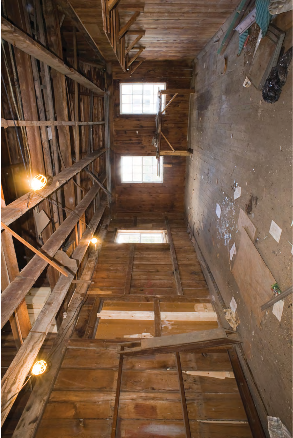
Photograph 21. Second floor south (rear) space. View to the southwest.
