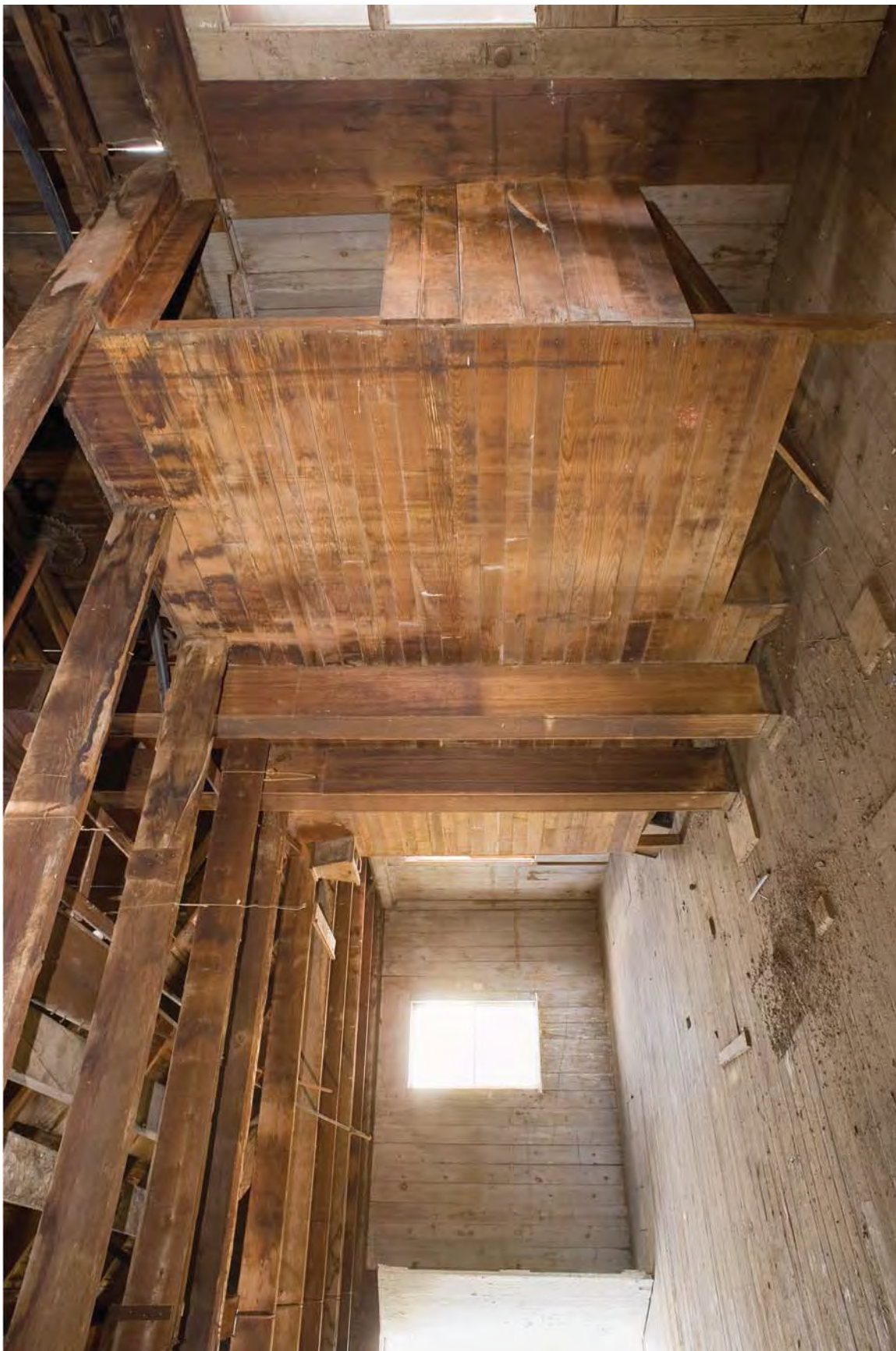
Photograph 22. Second floor front space, northeast corner. View to the northeast.
