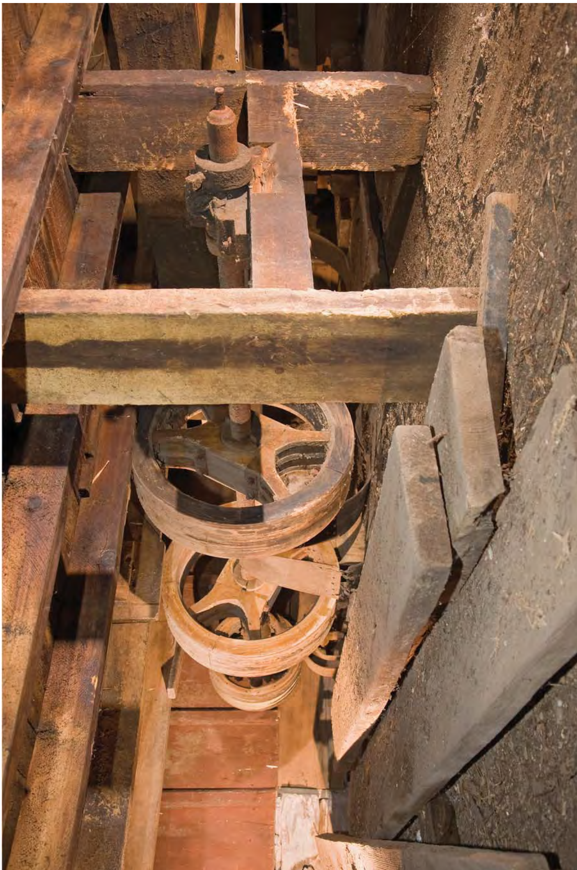
Photograph 17. Drive machinery, south end of first floor space "L." View to the northwest.
