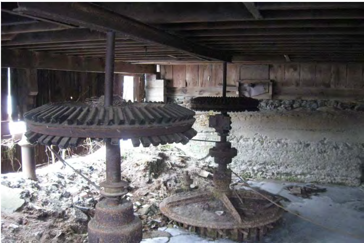
Photograph 8. Detail of the two intact water turbines, gearing, and shafting in situ beneath the extension denoted as section “K” in Figure 4.
