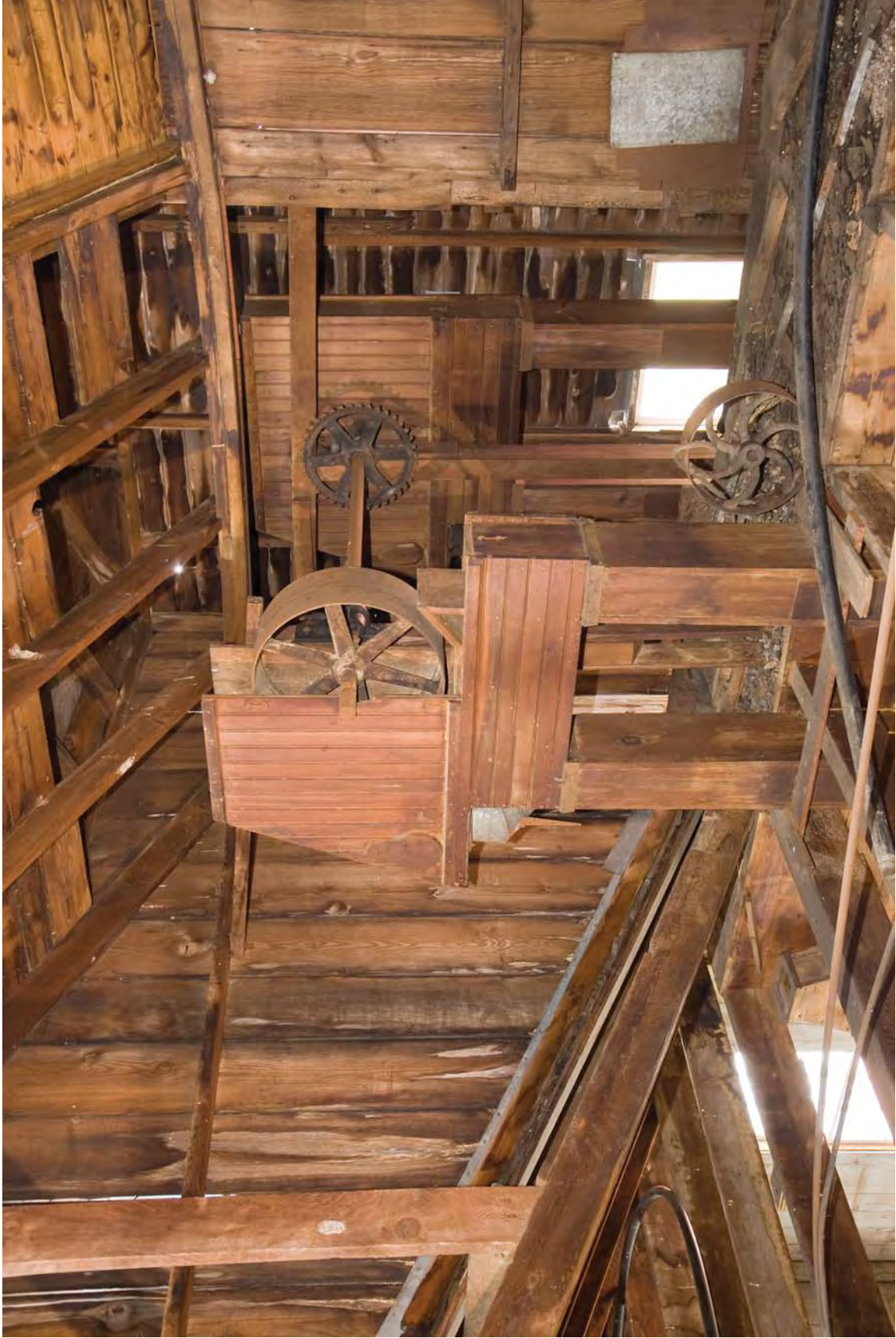
Photograph 27. Milling equipment in attic. View to the northeast.
