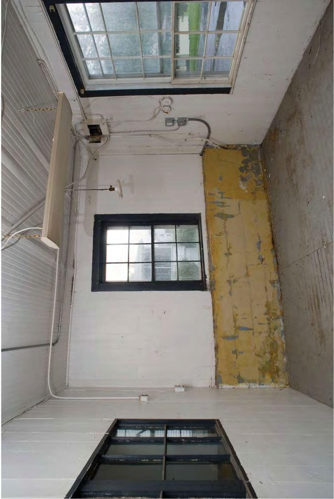
Photograph 20. First floor space, northwest corner. View to the northwest.
