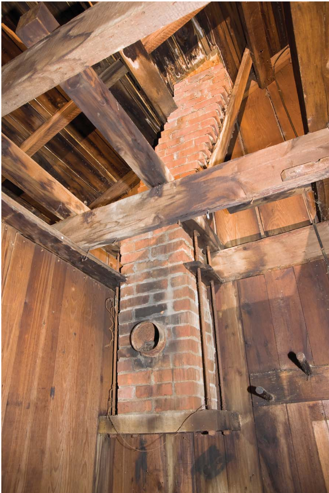
Photograph 24. Chimney, northwest corner. View to the northwest.
