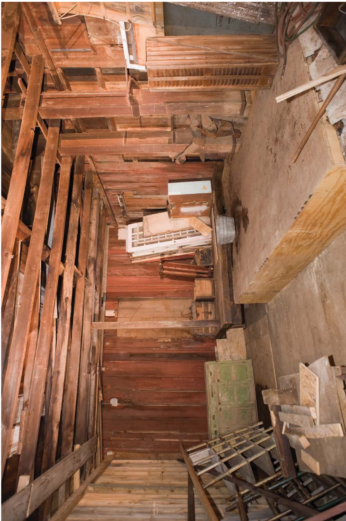
Photograph 18. First floor, east interior space "L." View to the south-southwest.
