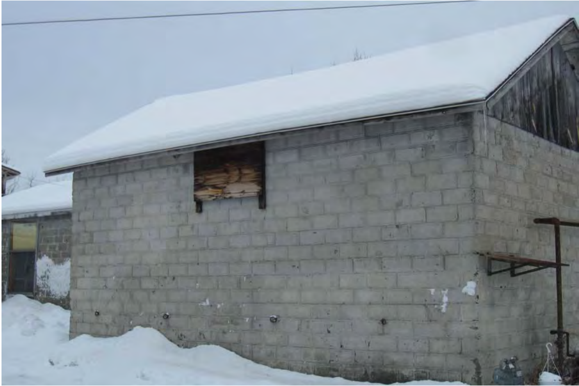
Photograph 5. View of concrete block building that partially housed a creamery operation until 1975. The steel rings set into the lower wall were used for hitching horses to the building.
