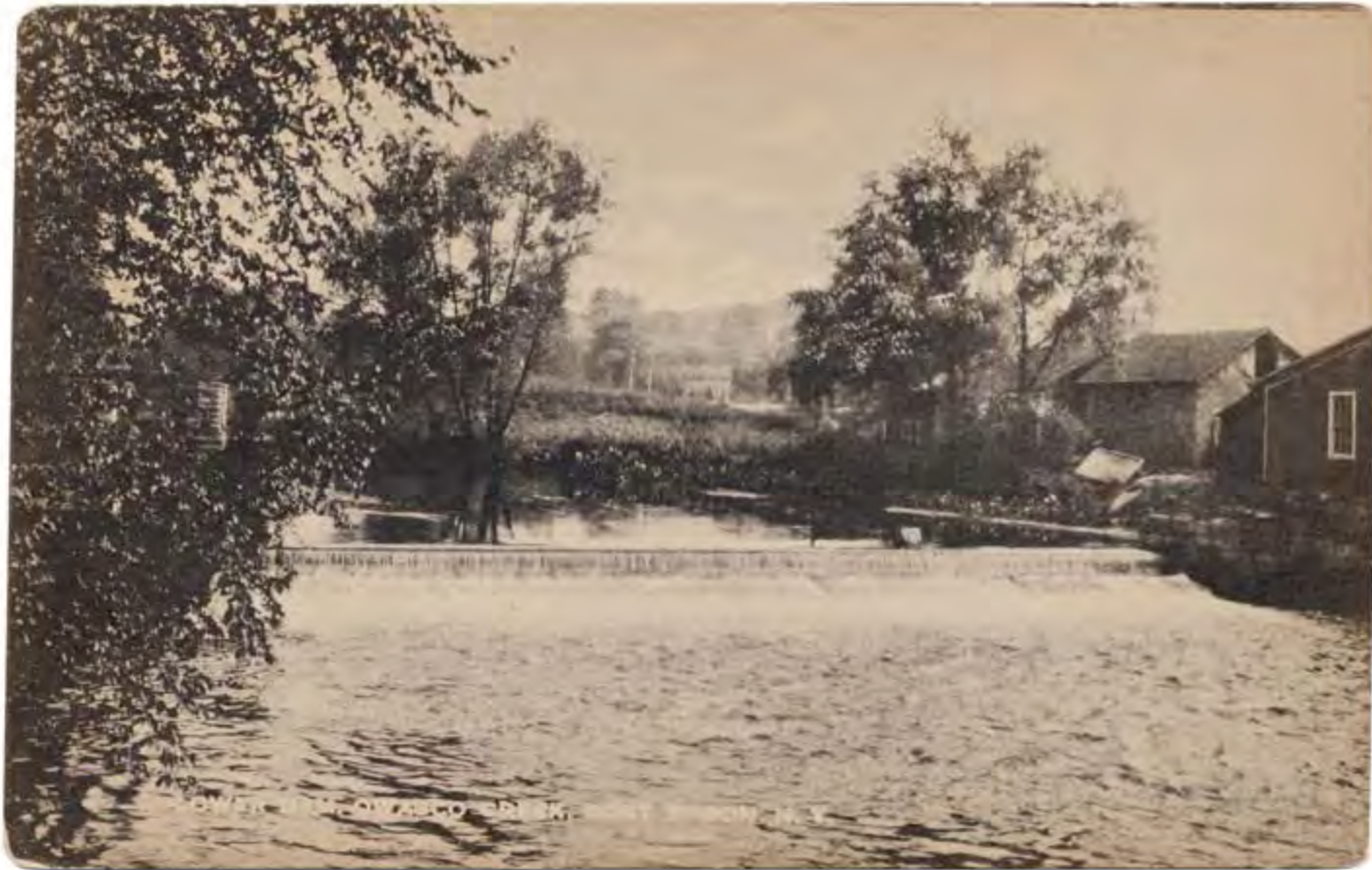
Figure 17. Undated view of the Owasco Outlet adjacent to the Project Area with the mill dam intact and an extension of the mill structure visible in the center right of the image that probably corresponds to section “E” in Figure 4. Note the masonry pier of the Erie Canal aqueduct in the image background. Image courtesy of Mike Riley.
